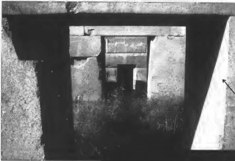
Fig. 2-9. Looking through the second temple. Arrow shows wall where Katrina took photo.
